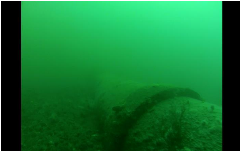
Figure 2 – Pipe Joint
