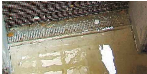
STEP SCREEN® with optimal bottom step design. The channel floor is flush with the top of the lowest step.
