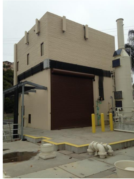
Odor Control Scrubber Tower
