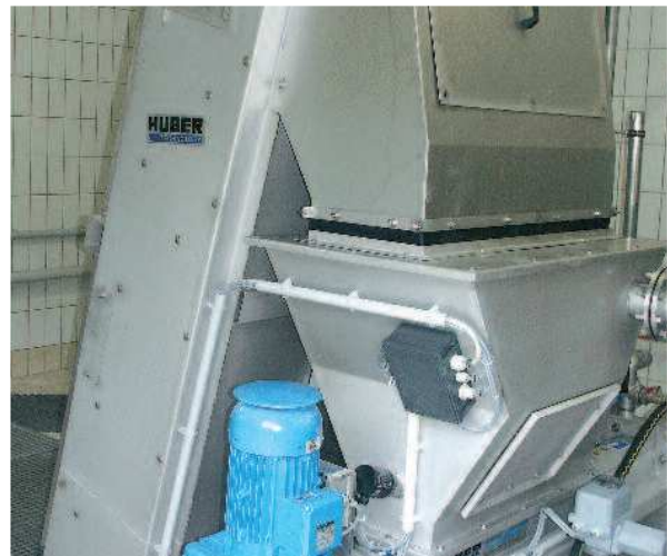
Rear view of a HUBER RakeMax® Screen with subsequent Wash Press WAP/SL
