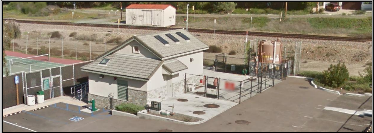
Figure 1 - 21 st Street Pump Station, City of Del Mar
