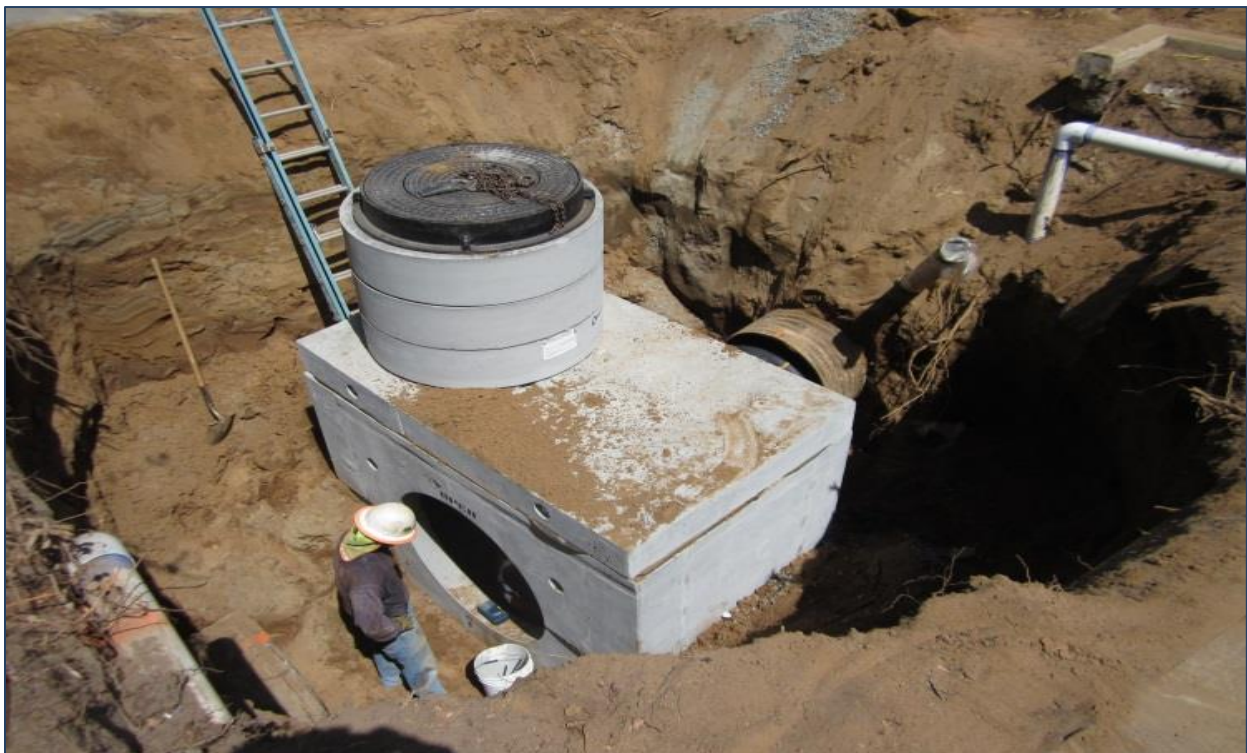
Storm Water Diverter Installation
