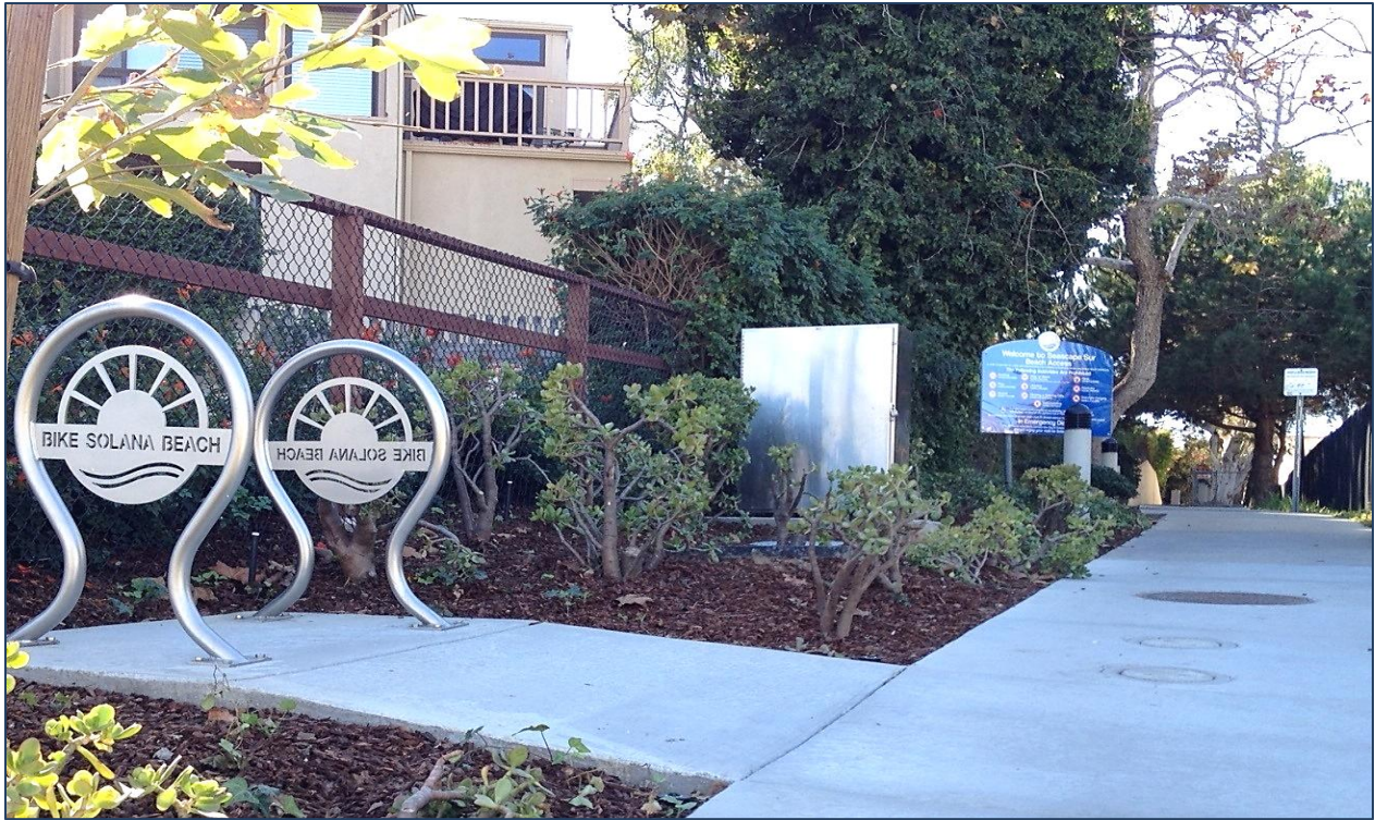
Completed Storm Water Diverter Site
