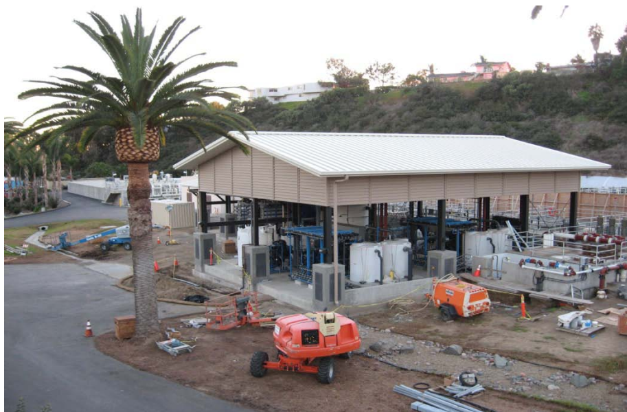
Advanced Water Treatment project under construction.
