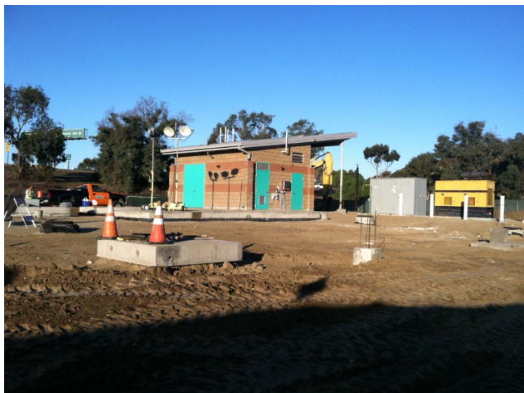
New Olivenhain Pump Station under construction.
