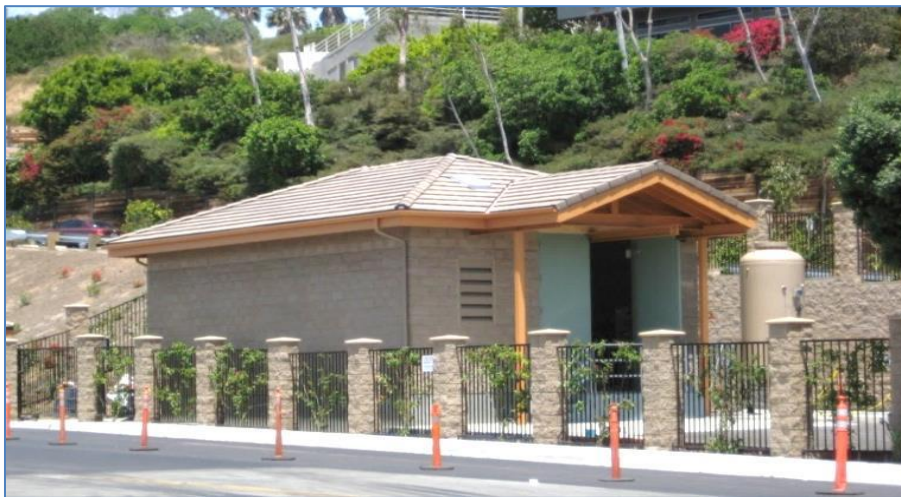
Eden Gardens Pump Station
