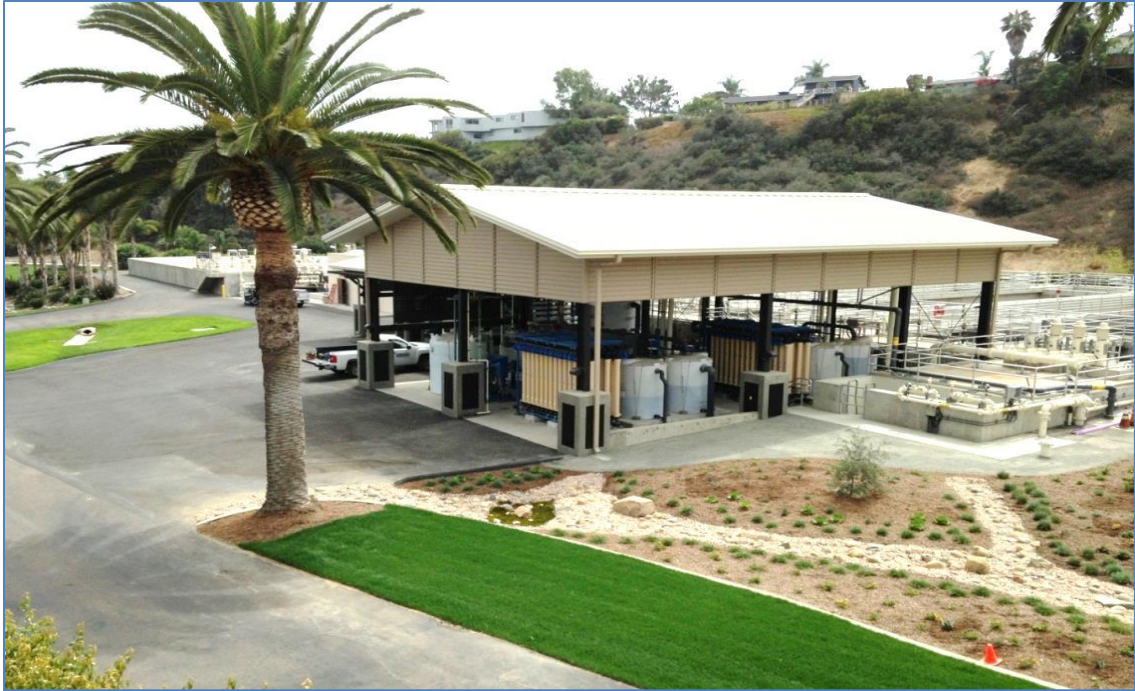
Advanced Water Treatment Facility
