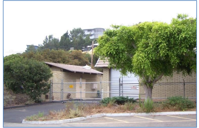
Cardiff Pump Station
