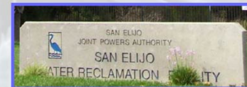
The plant provides the community with a source of recycled water for a variety of uses.
