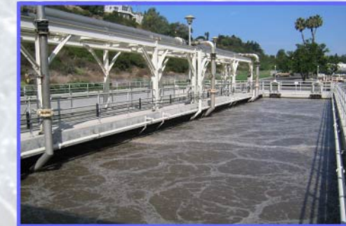
Wastewater as it starts through secondary treatment at the San Elijo Water Reclamation Facility.
